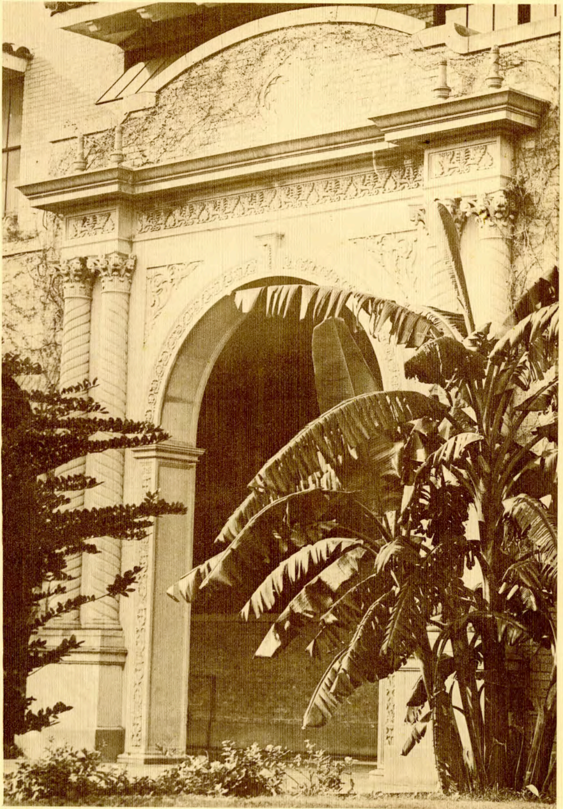
The Front Doorway
