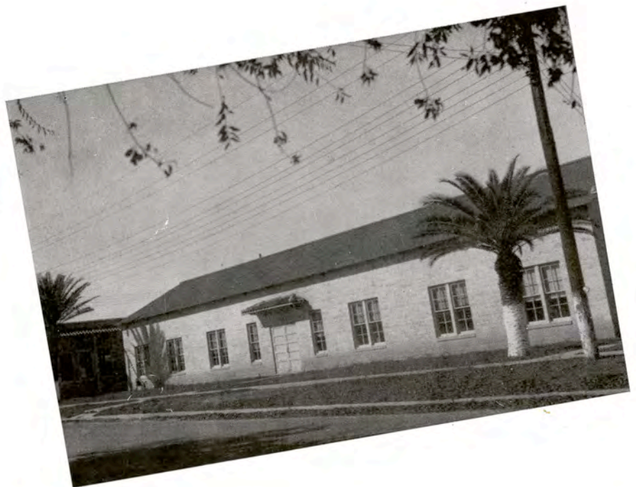
Natural Gas Engineering Building
