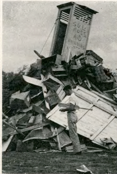
Building the Bon
