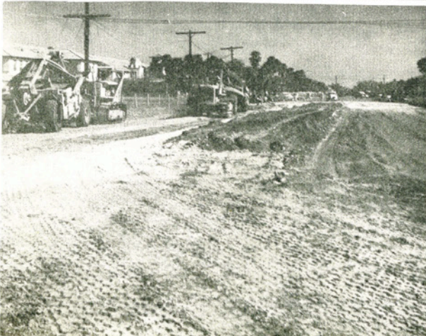
construction work around the campus . . .
