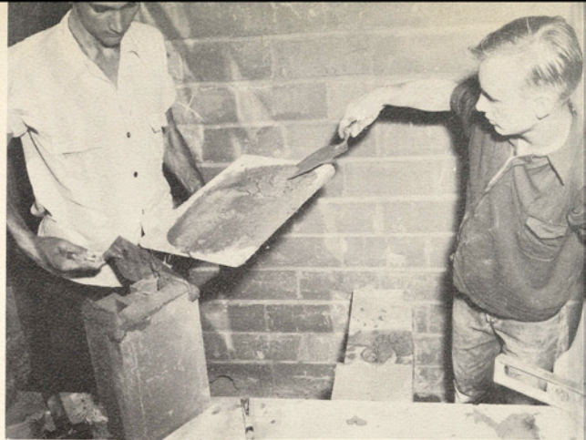
Work on the Ag Engineering building was being completed.
