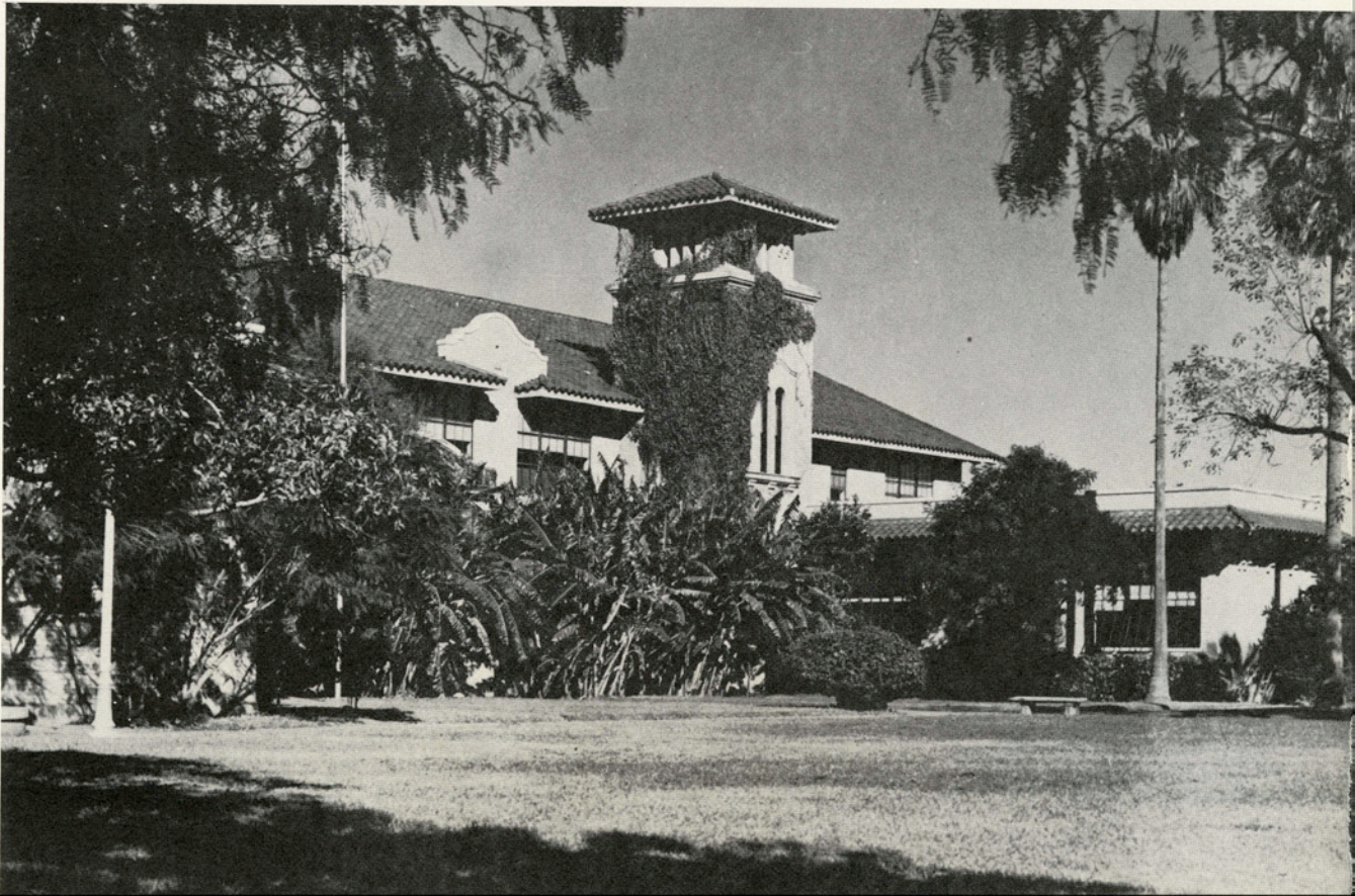
Old Administration Building
