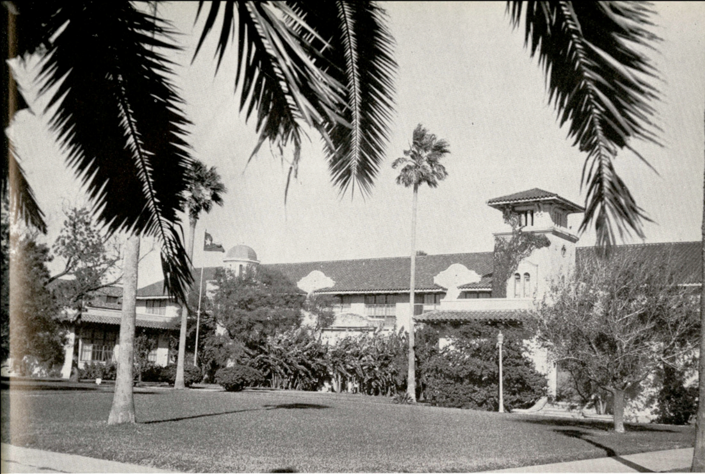
OLD ADMINISTRATION BUILDING
