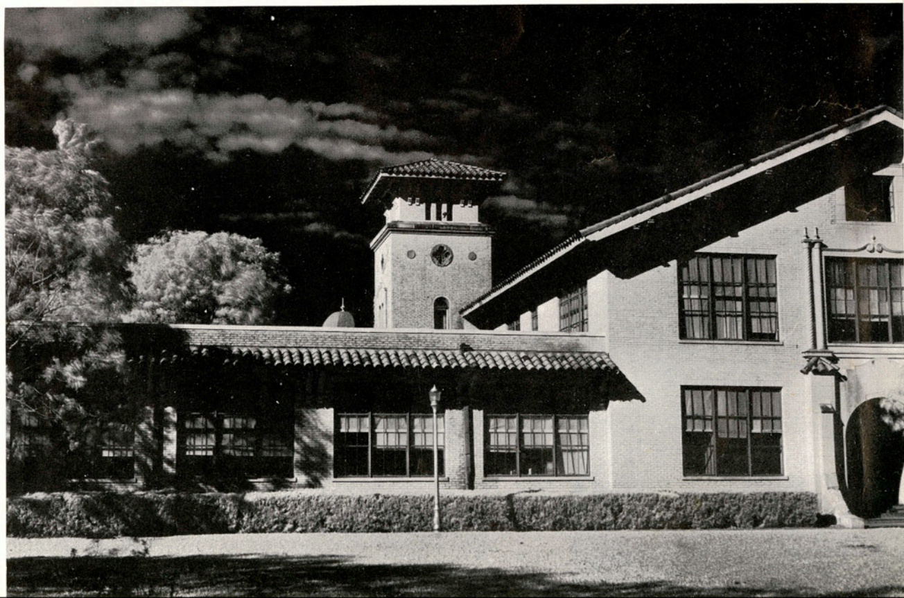
OLD ADMINISTRATION BUILDING
