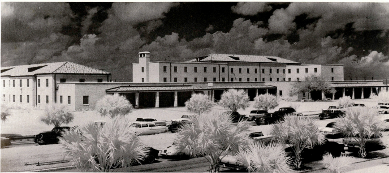
LEWIS AND ECKHARDT HALLS
