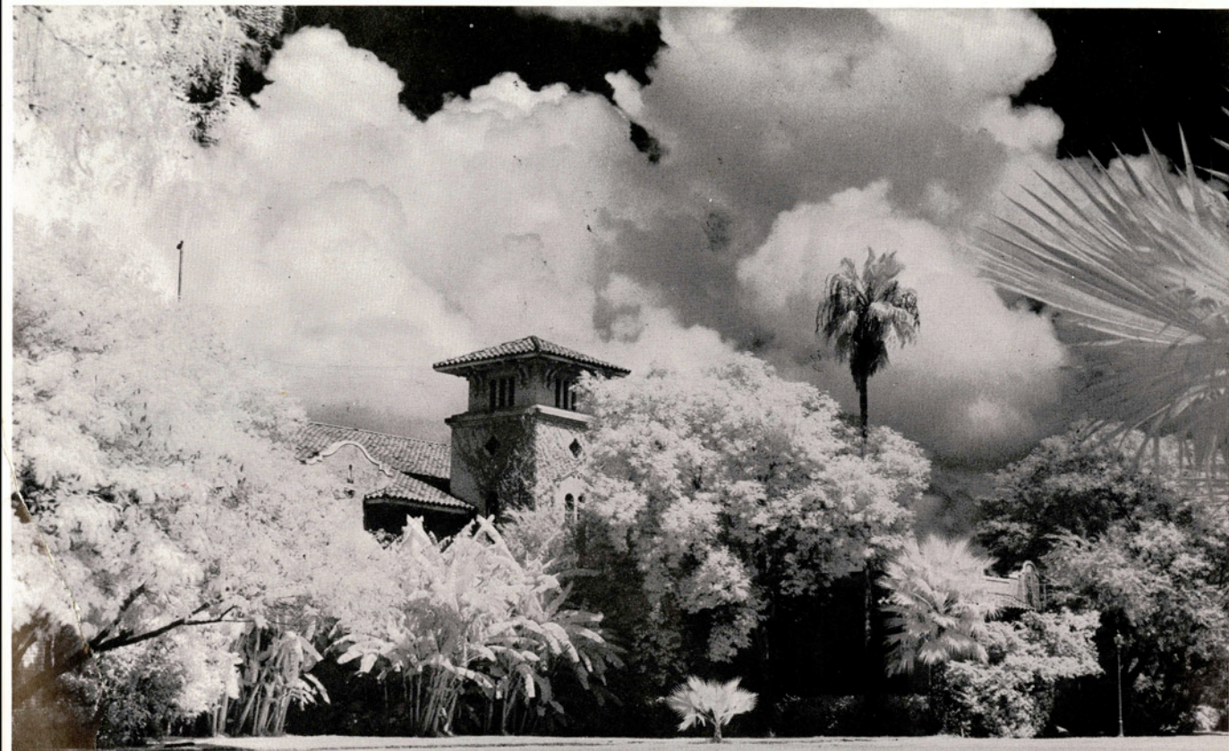
OLD ADMINISTRATION BUILDING
