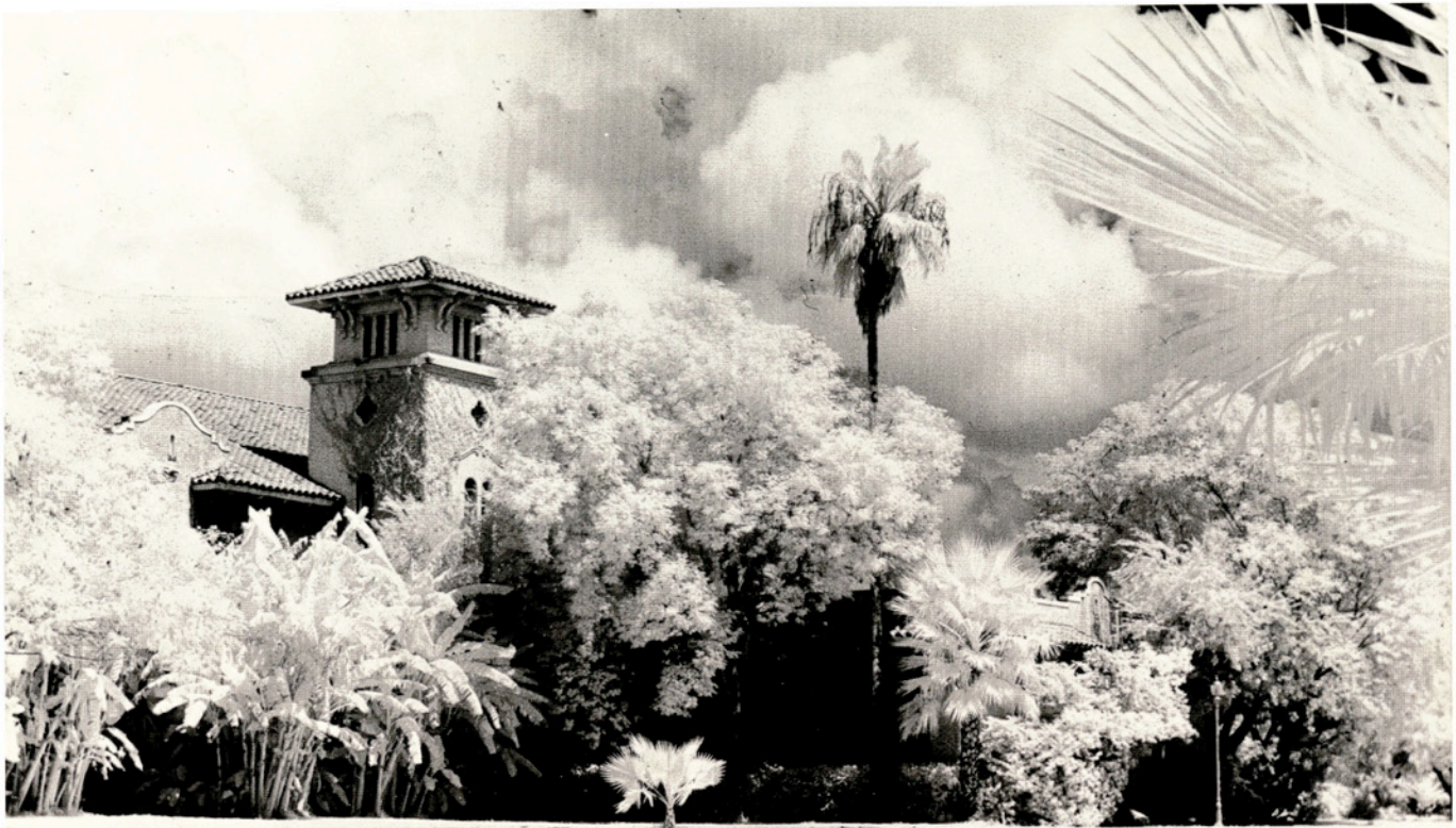
OLD ADMINISTRATION BUILDING
