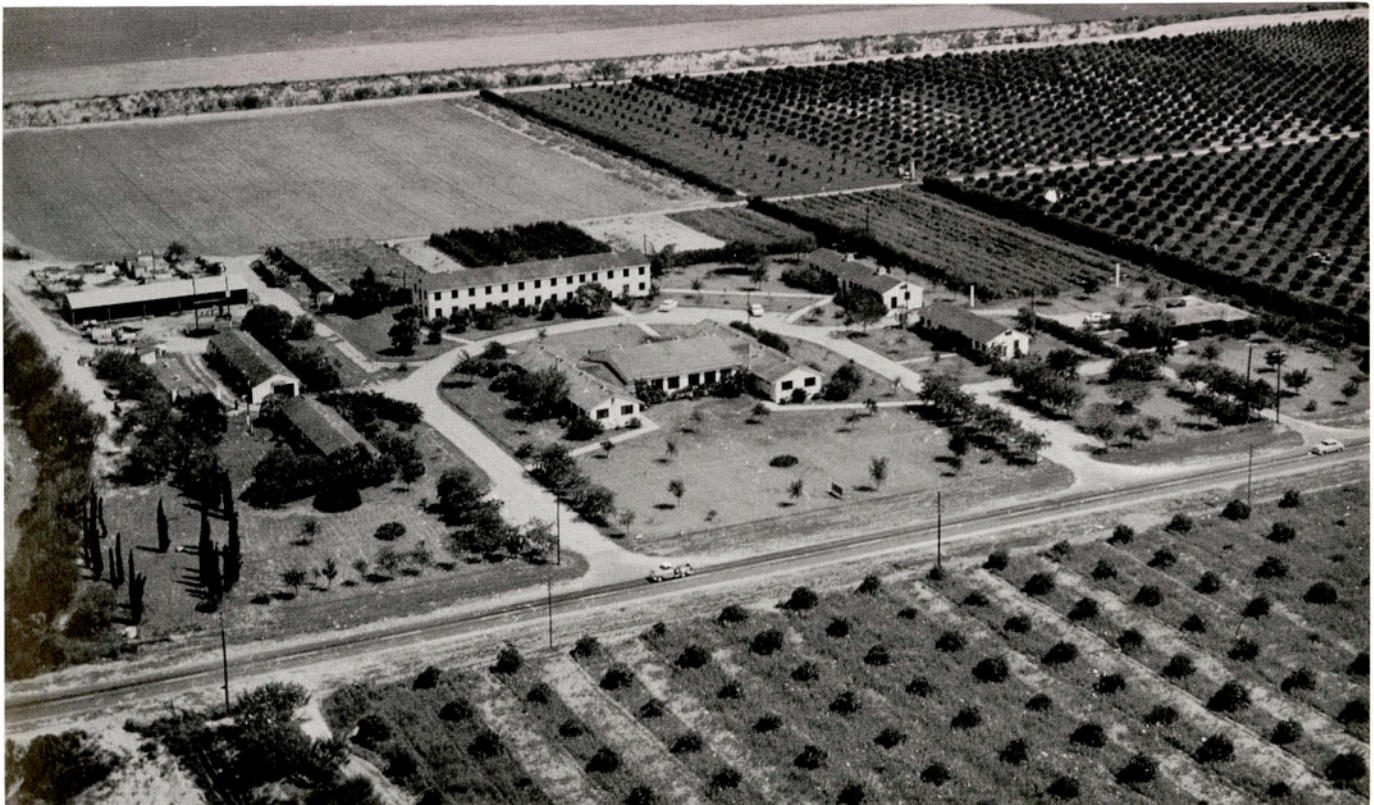
Aerial view of part of A&I Citrus and Vegetable Training Center
