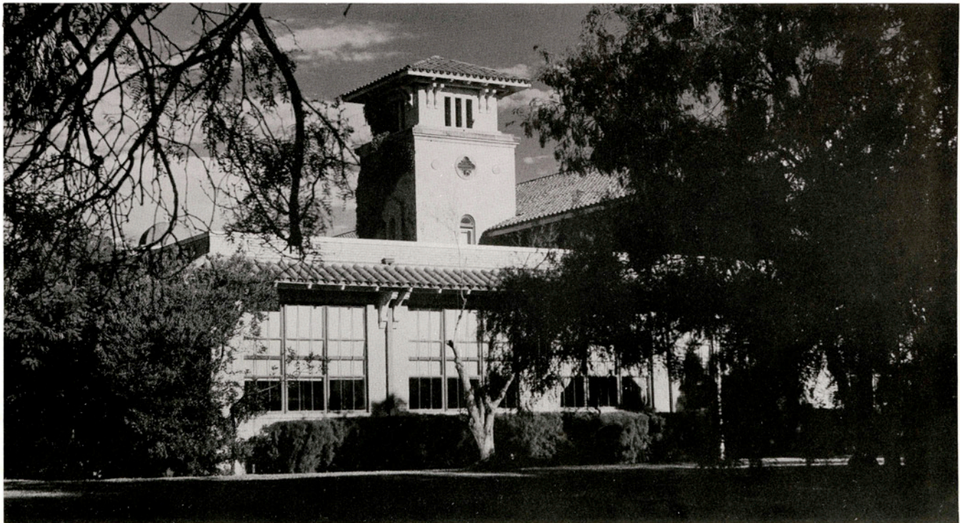
Old Administration Building
