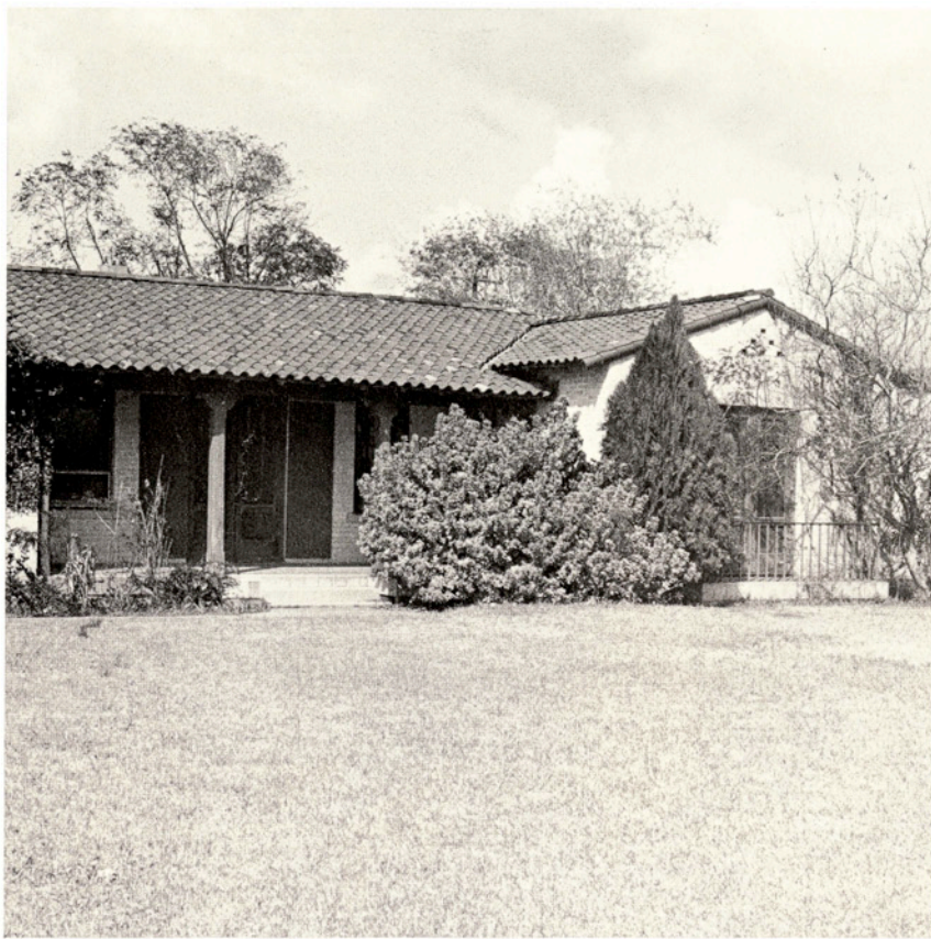
The A&I Farm Cottage, built in 1934, will give way to the new as a dorm is erected on the ground where it now stands. The cottage, south of Martin Hall, has housed four faculty families in its 35-year history. Now empty, the cottage awaits its eventual destruction or removal.
