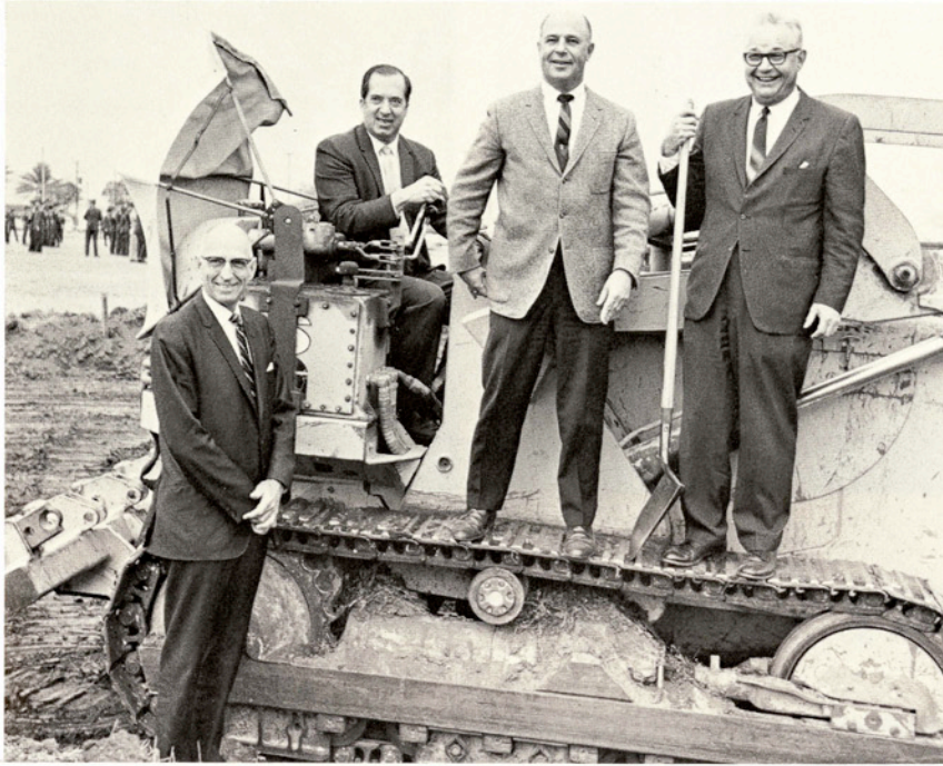
With a 20 per cent enrollment increase, eight new buildings are in various stages of planning for A&I. An Industrial Arts building, costing approximately $346,193, was started this year. At the groundbreaking ceremonies were Dean Robert Rhode; A. F. Gross, IA department chairman; Dr. John W. Glock, Dean of Teacher Education; and President James C. Jernigan.
