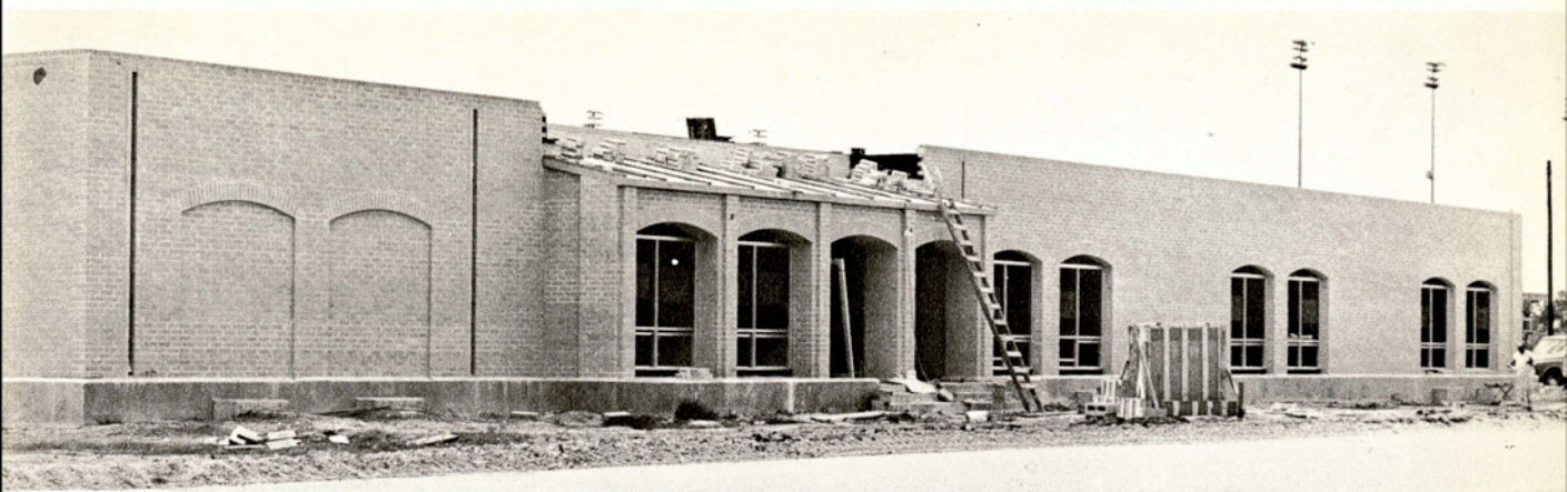
The new Industrial Arts building was completed in time for spring semester classes.
