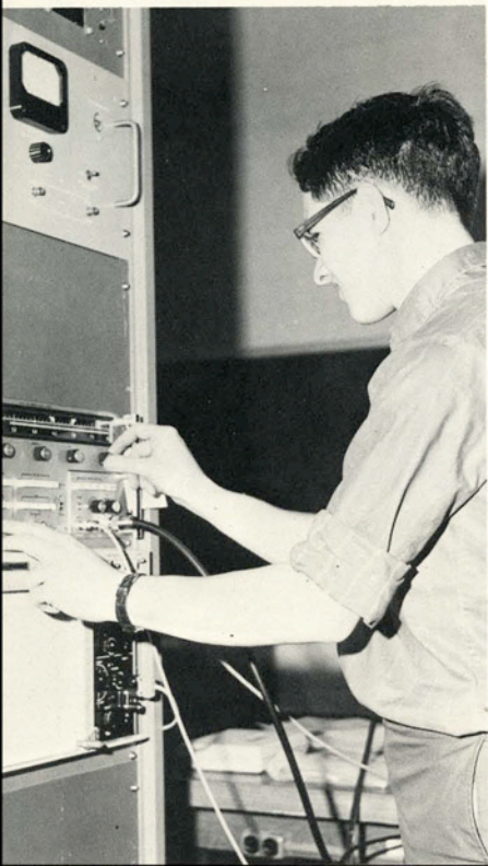
John Phalen, graduate assistant in electrical engineering, sets up an experiment in the micro-wave laboratory. The experiment is a feasibility study in determining moisture content of grain by micro-wave power.
